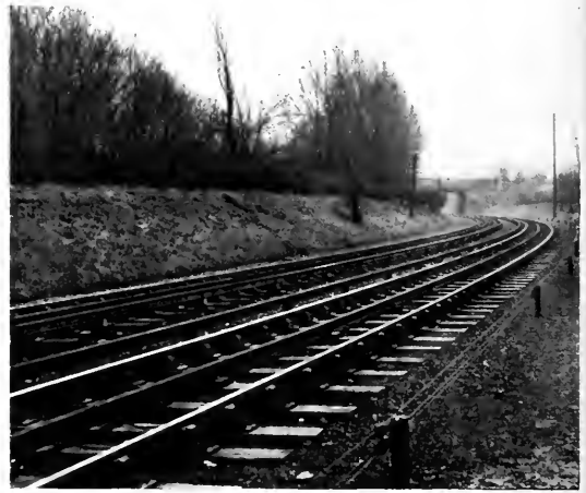
FIG. 1.—VIEW SHOWING THIRD AND FOURTH RAILS.
